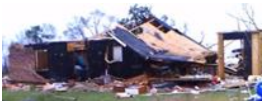
Fig. 2 This image was used on the survey. The damage shown is EF-2 damage from the Jones County, MS tornado of 20 December 2007
